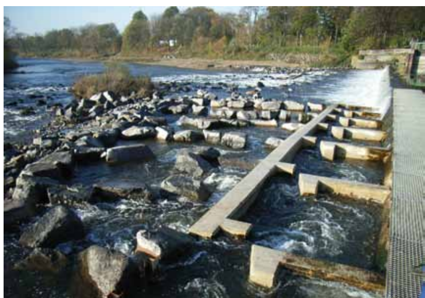
Fishpass and fish monitoring station
